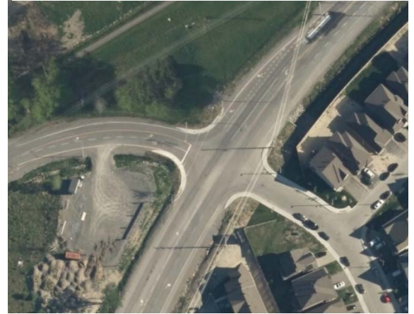
Figure 1 - Fallowfield Road & O’Keefe Court / Cobble Hill Drive intersection
