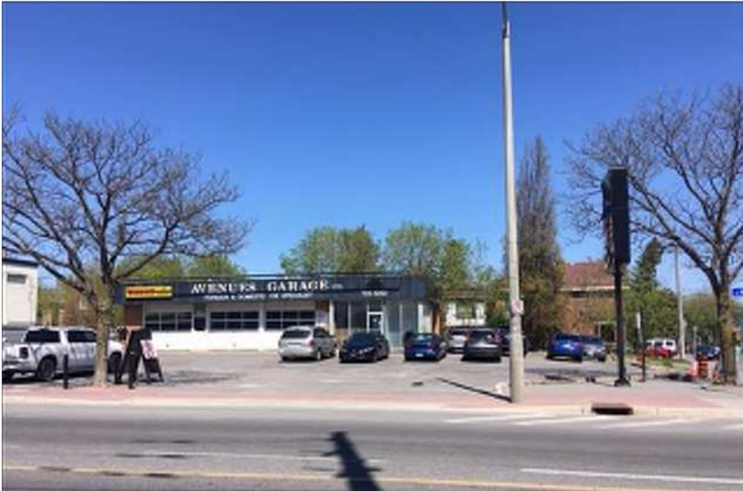
Photograph 1: View of the former automotive repair garage at 319 Richmond Road.
