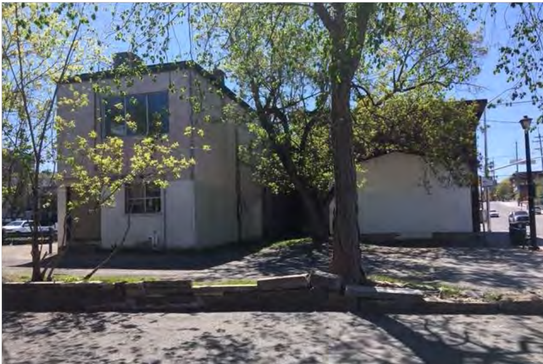
Photograph 4: North view of 325 and 327 Richmond Road, looking towards Richmond Road.
