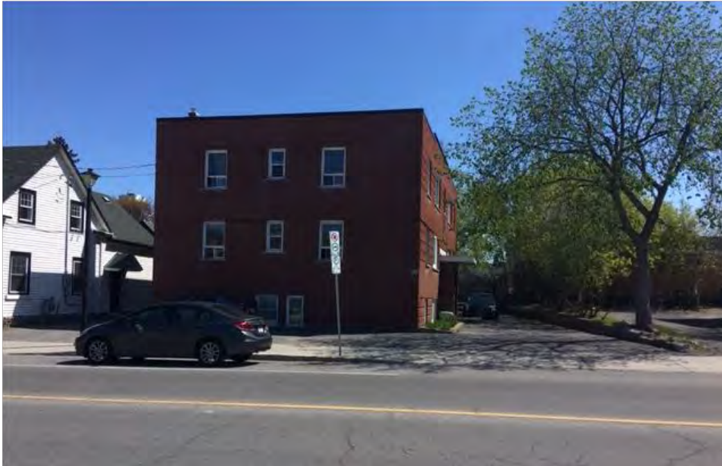
Photograph 5: View of the residential apartment building at 381 Churchill Avenue.
