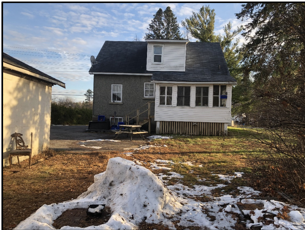
Photograph 2: Rear view of subject property, looking south.
