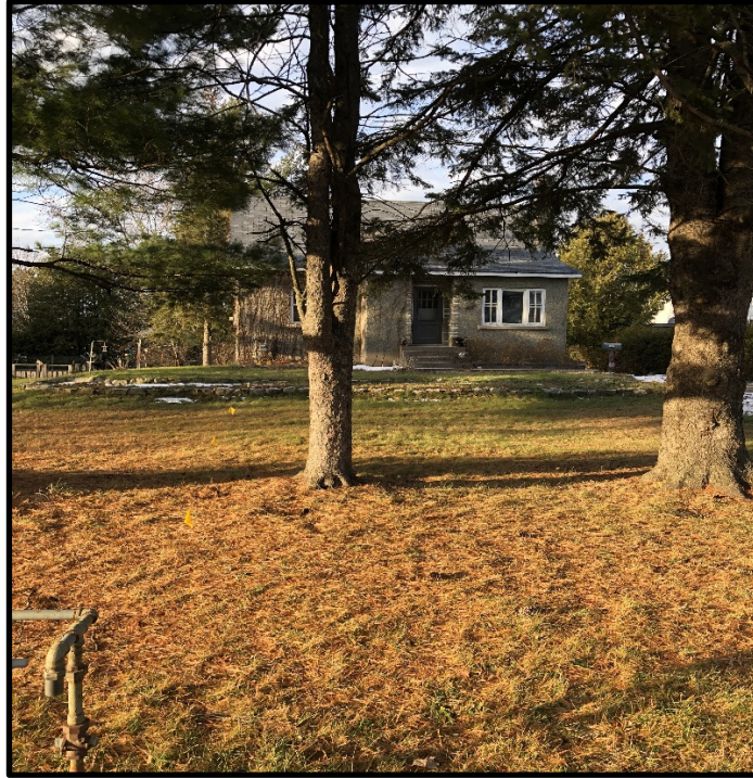
Photograph 1: Front view of the subject property, looking north.
