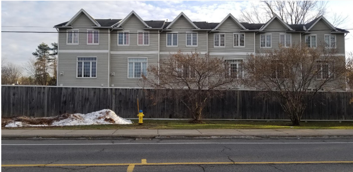
The view to the south and the rear yards of 6-unit townhouse row on Scotland Private.
