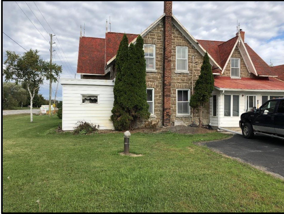
Photograph 5: View of the residential dwelling, looking north.
