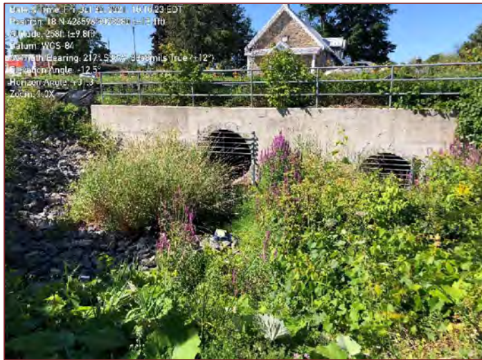
Site Photograph 9 – Inlet for Tributary 4
