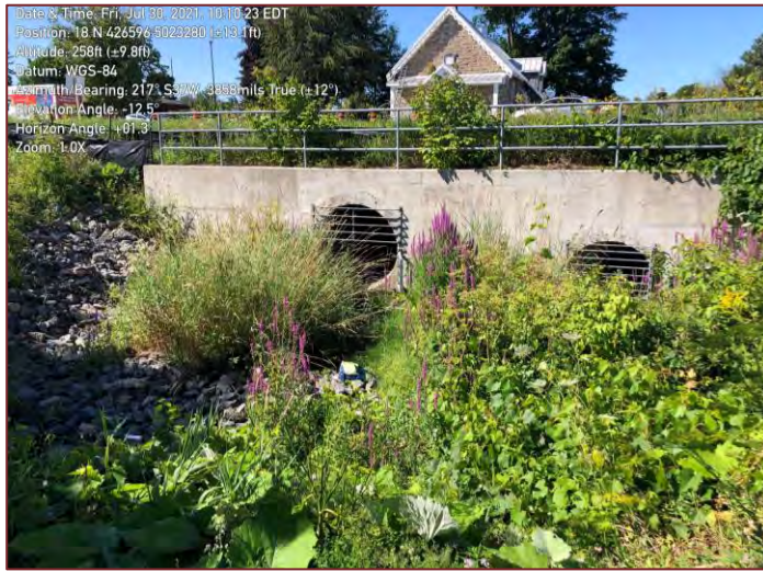
Site Photograph 9 – Inlet for Tributary 4
