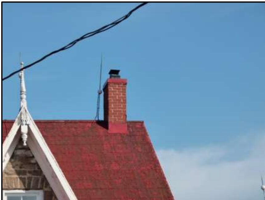
Photograph 30: 910 March Road (Building #1) chimney with metal cap (August 14 th , 2017).
