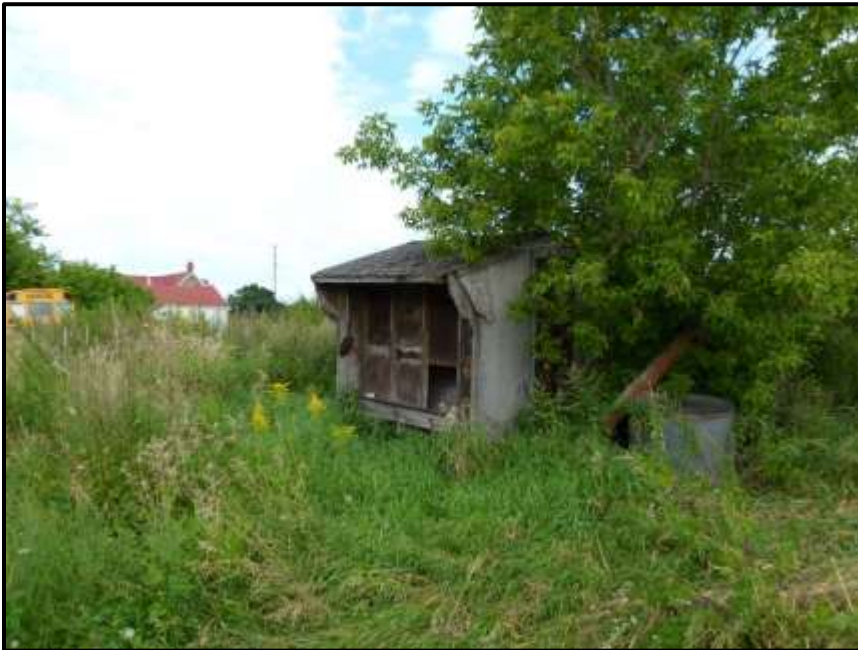
Photograph 28: Building #9 – no Barn Swallow nests were noted (August 14 th , 2017).
