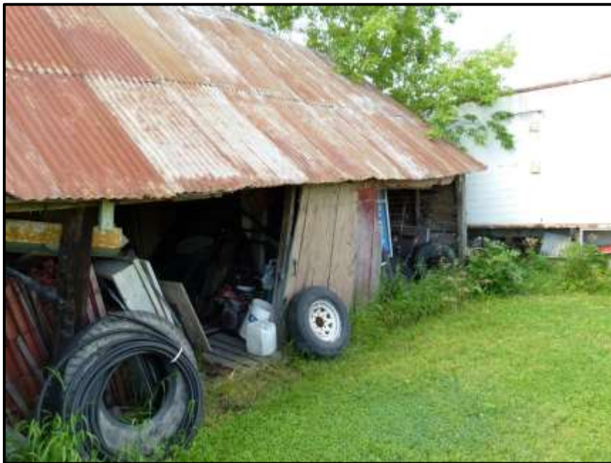
Photograph 22: Building #4 – one (1) intact and one (1) degraded Barn Swallow nest were noted (August 14 th , 2017).
