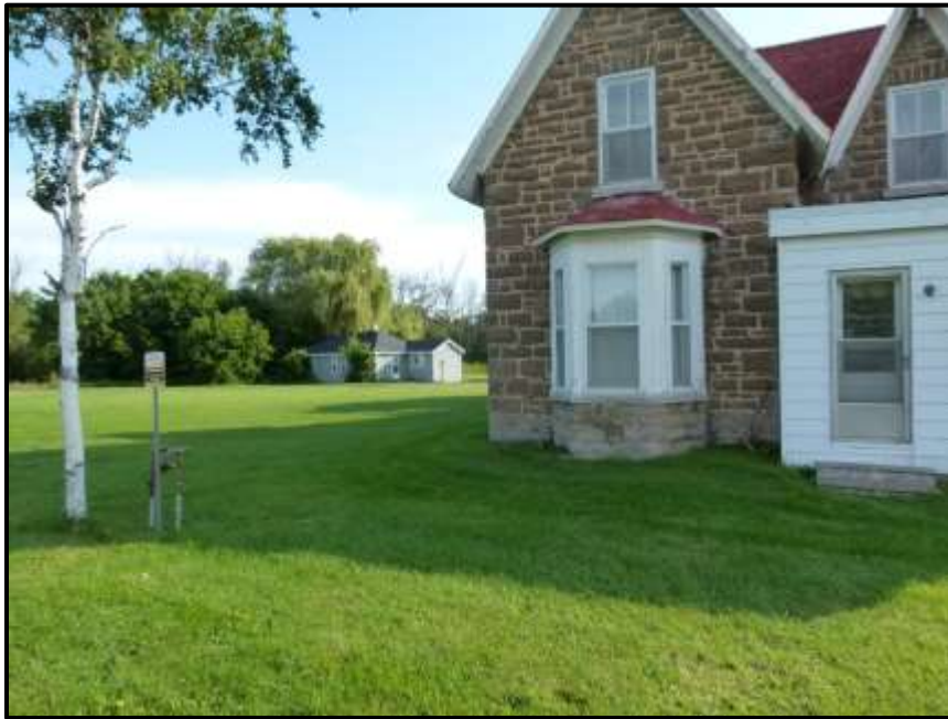
Photograph 1: Looking northeast at 910 March Road (Building #1) (foreground) and 920 March Road (Building #5) (background). Note the manicured lawn in the western part of the Site (August 14 th , 2017).
