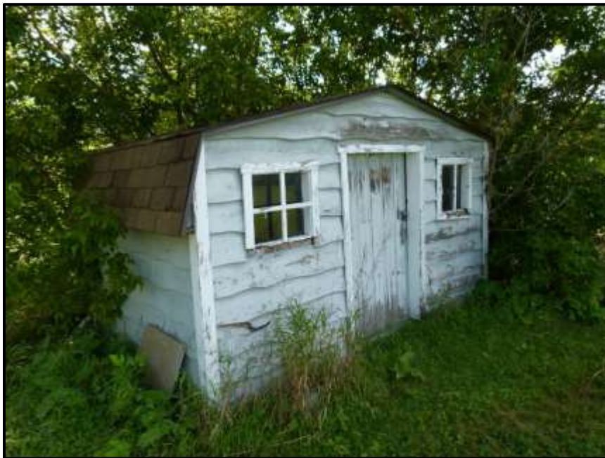
Photograph 24: Building #6 – no Barn Swallow nests were noted (August 14 th , 2017).
