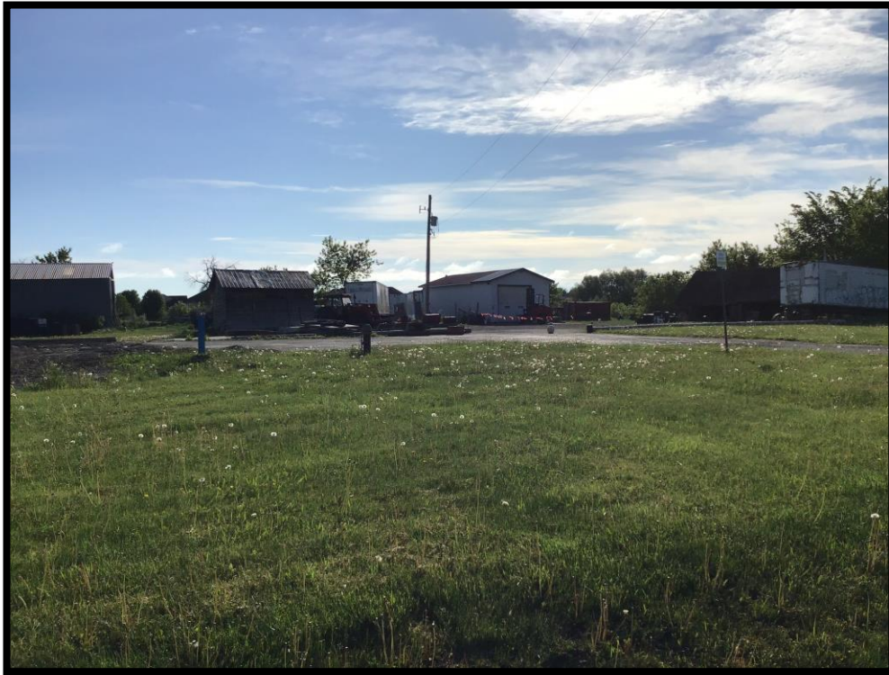
Figure 5: Overview of depot outbuildings and lawn fronting March Road (PA1170-02E).
