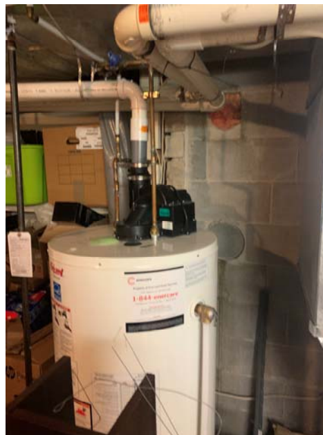
View of existing hot water tank
