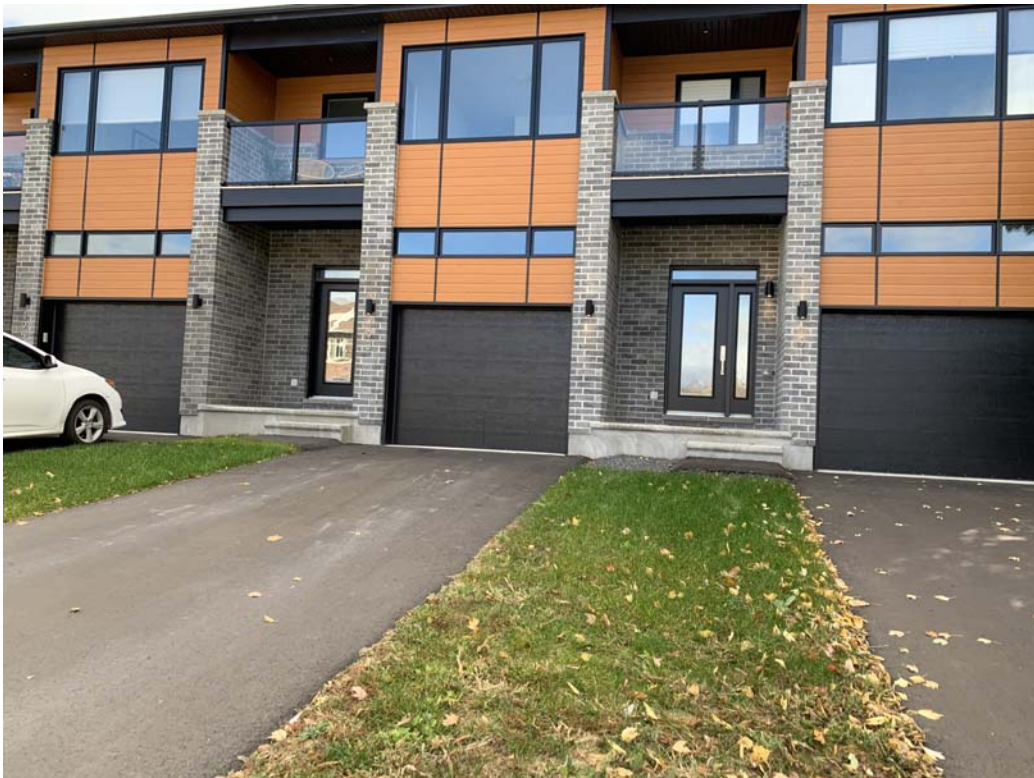
New residential dwelling located northwest of the site
