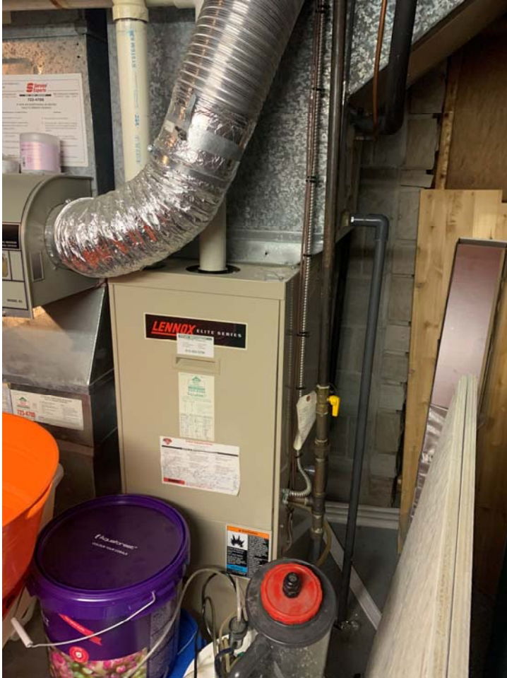
View of existing furnace and humidifier within basement of dwelling
