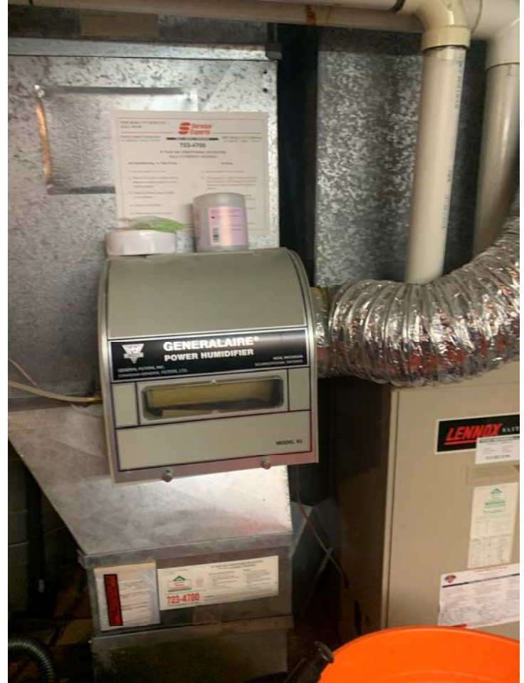
View of existing furnace and humidifier within basement of dwelling
