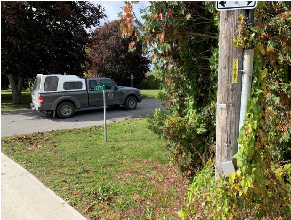
View of hydro pole at southeast corner of property
