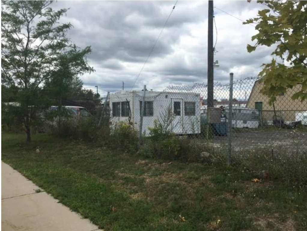
Photo 11: Fuel AST located on the automotive garage property at 4065 Bank Street.
