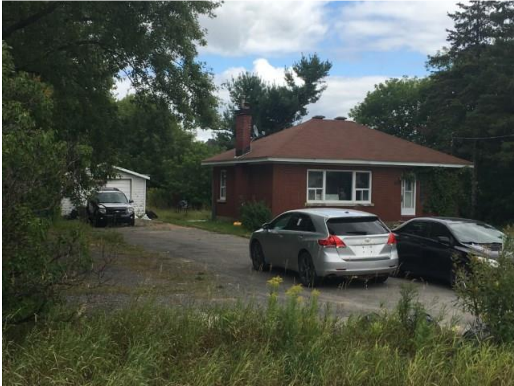
Photo 7: Photo of the fill and vent pipes observed on a residential house south of the Site at 4695 Bank Street.
