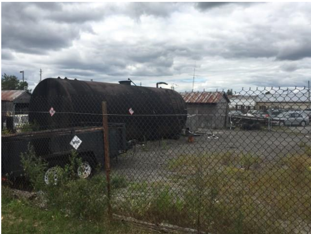
Photo 4: Photo of the tar or asphalt AST on the former asphalt company property north of the Site at 4603 Bank Street.
