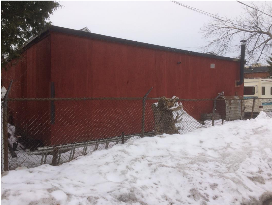
Photograph 1: Adjacent private automotive service garage and exterior AST.
