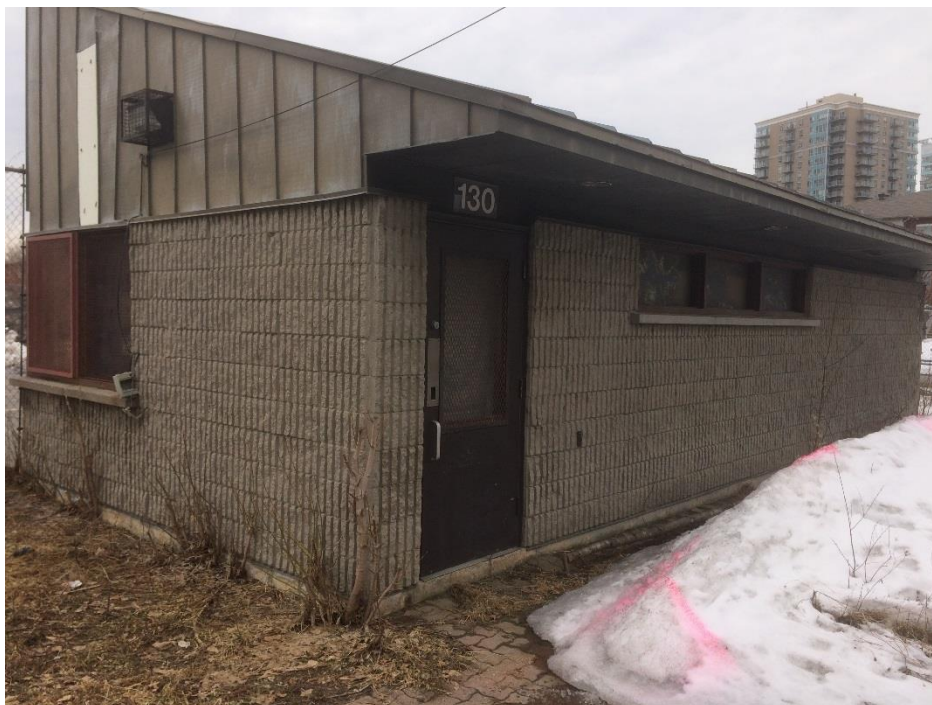
Photograph 4: Storage building near parking area. No access was provided to the interior of this building.
