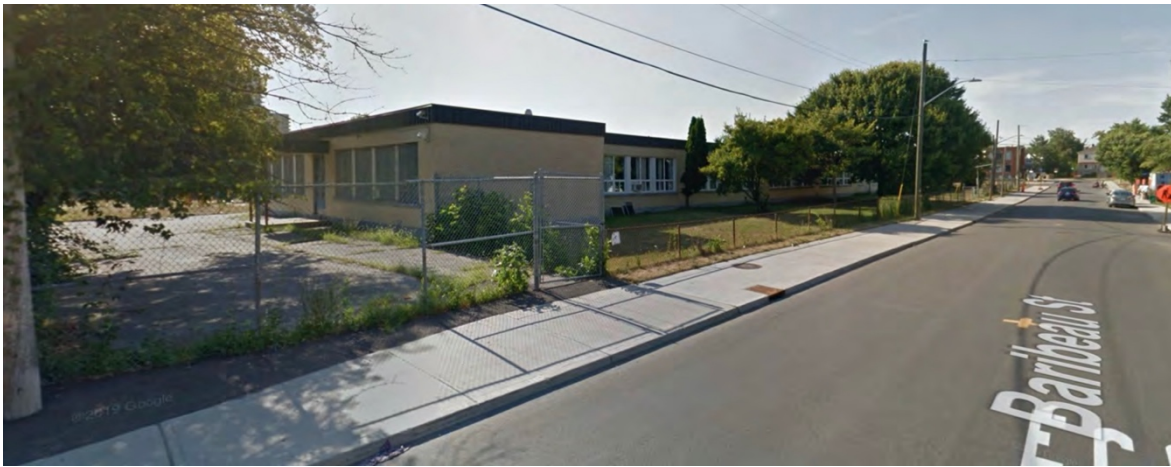
Figure 4: View of site from the west property line on Baribeau Street
