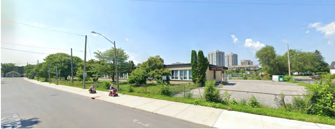
Figure 3: View of site from Baribeau, looking north west into the site
