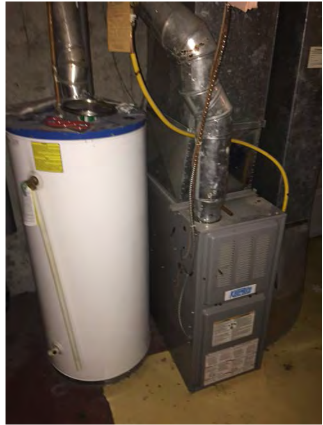
Example of natural gas powered furnace and water heater at 16 and 18 Dunbar Court
