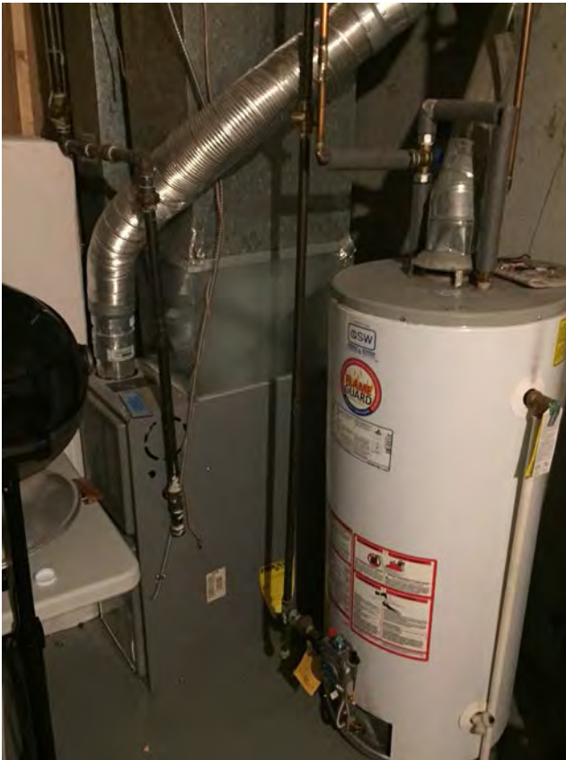
Example of natural gas powered furnace and water heater at 16 and 18 Dunbar Court
