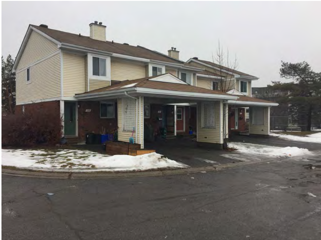
Front view of site northeast
