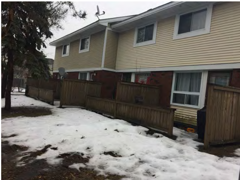
Rear view of site facing east
