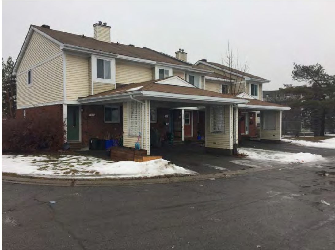
Front view of site northeast
