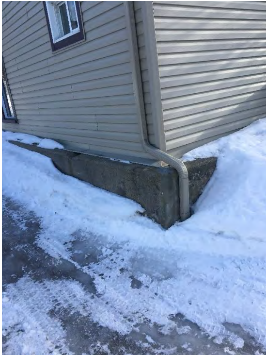
Roof drainage (east)
