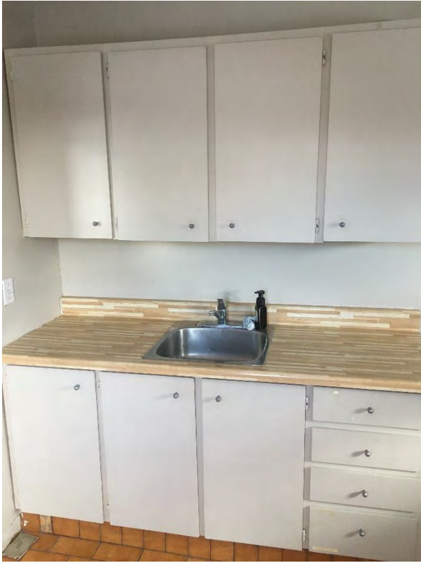
Kitchen (2 nd floor)
