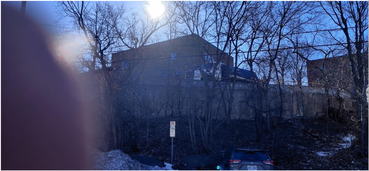
Photograph Plate 17: View of the southeast of the Site from Danforth Avenue. Location of Laundry Land (dry cleaning shop).
