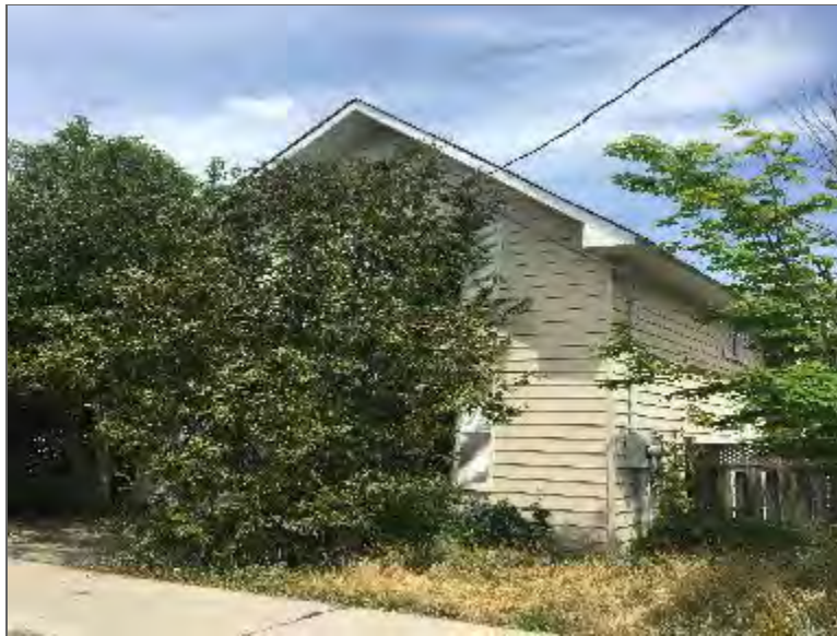
Photo 4 – Site Building (west elevation).
