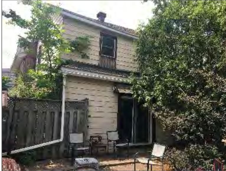
Photo 3 – Site Building (east elevation).
