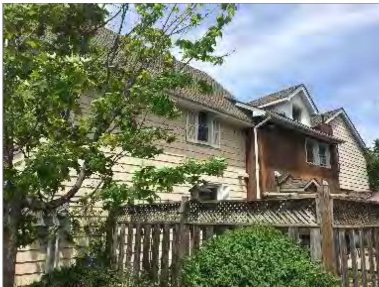
Photo 2 – Site Building (south elevation).
