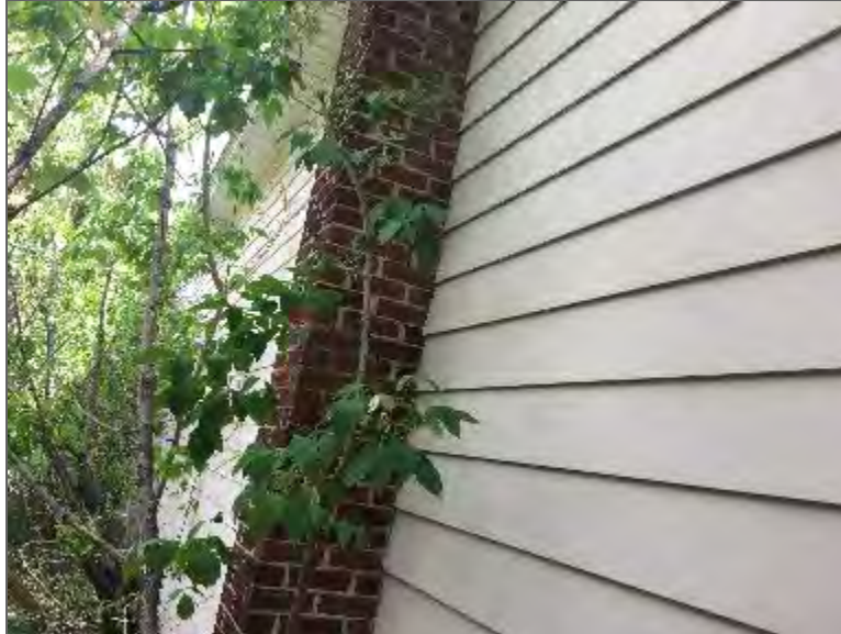
Photo 1 – Site Building (north elevation).
