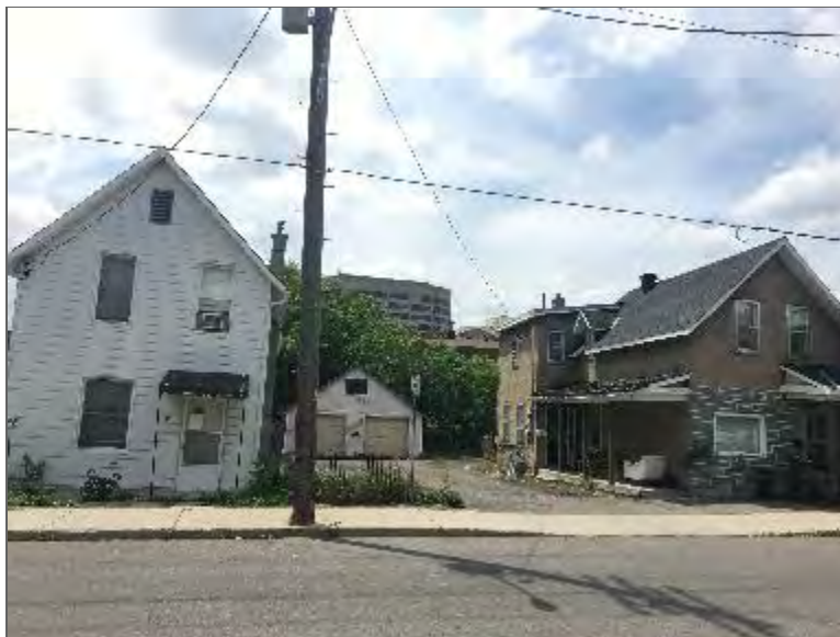
Photo 8 – Properties located west of the Phase One Property (with off-Site pole-mounted transformer (PCA) evident).
