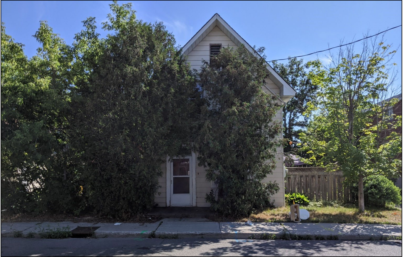
Figure 12. Existing frontage at 161 Hinchey Avenue.
