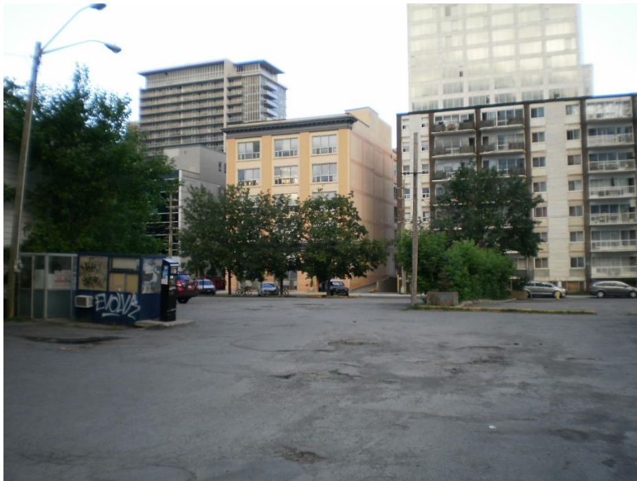
Photo 1 – Central and west portions of the site, with planted Norway maples in the rear on the south side of Nepean Street. View looking north from north of Lisgar Street
