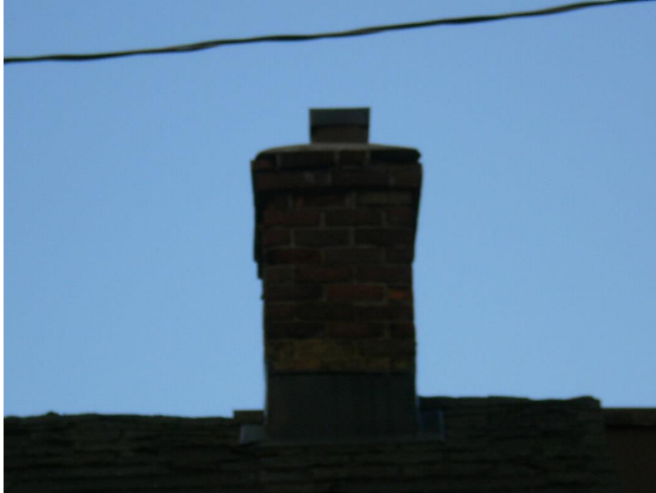
Photo 4 –Chimney on the remaining residence in the southwest portion of the site.
