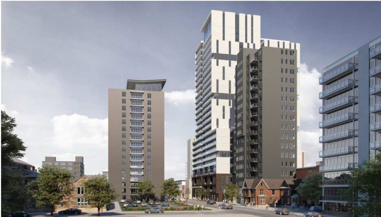
Figure 15: Perspective rendering of Lisgar looking west provides context. The facades of the first three storeys treated with a dark-brown brick reference the material and scale of the existing neighbouring buildings. Source: Graziani & Corazza Architects 2020
