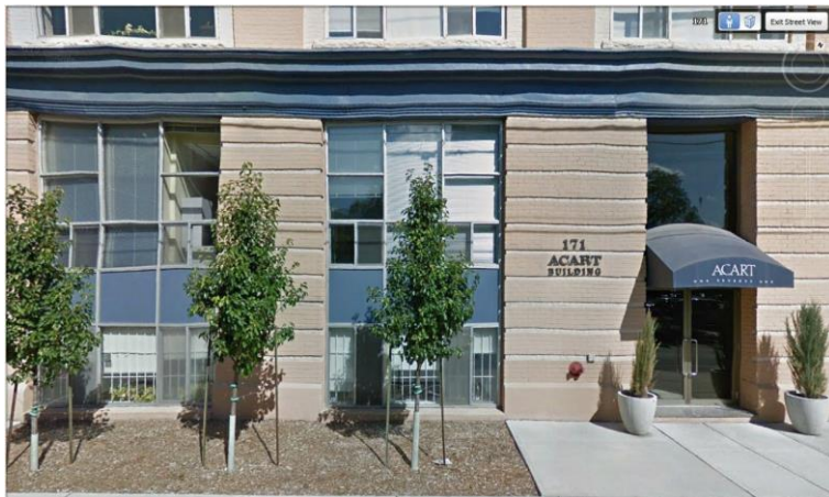
Figure 8: Context view of a six-storey development on Nepean Street across from the proposed development. Note the building is set 3.0m from the property line. Note the differing architectural and material treatment and the horizontal band, which in the absence of a step back visually at the street level forms a podium.
