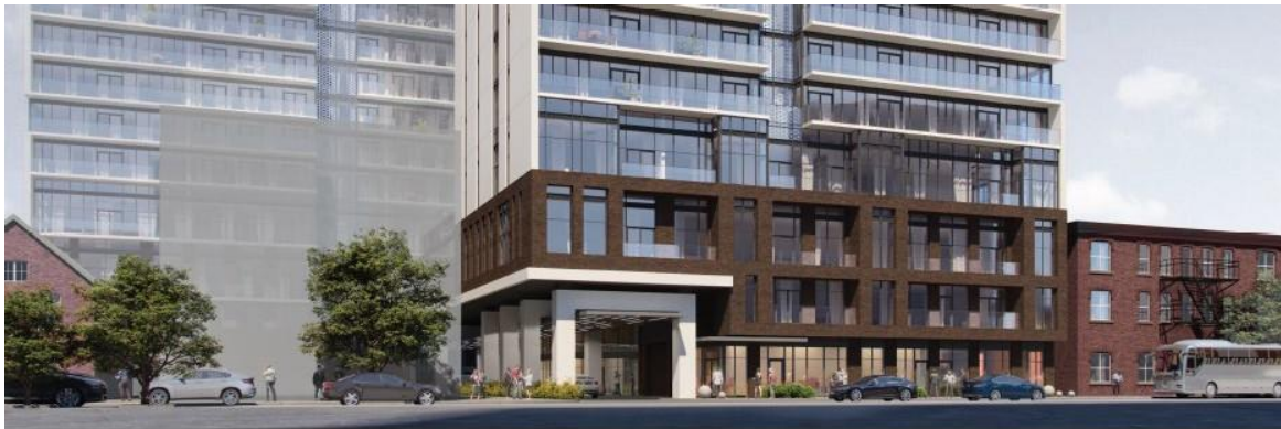
Figure 19: The perspective rendering of the Nepean streetscape features a two storey colonnaded drive isle that helps ground the tower. Carrying the glazing around the north and south facades at the 4 th floor might define the podium more distinctly. Source: Graziani & Corazza Architects 2021.
