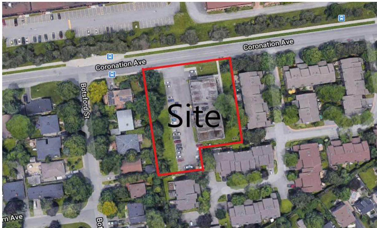
Figure 1: Aerial View of Proposed Development
