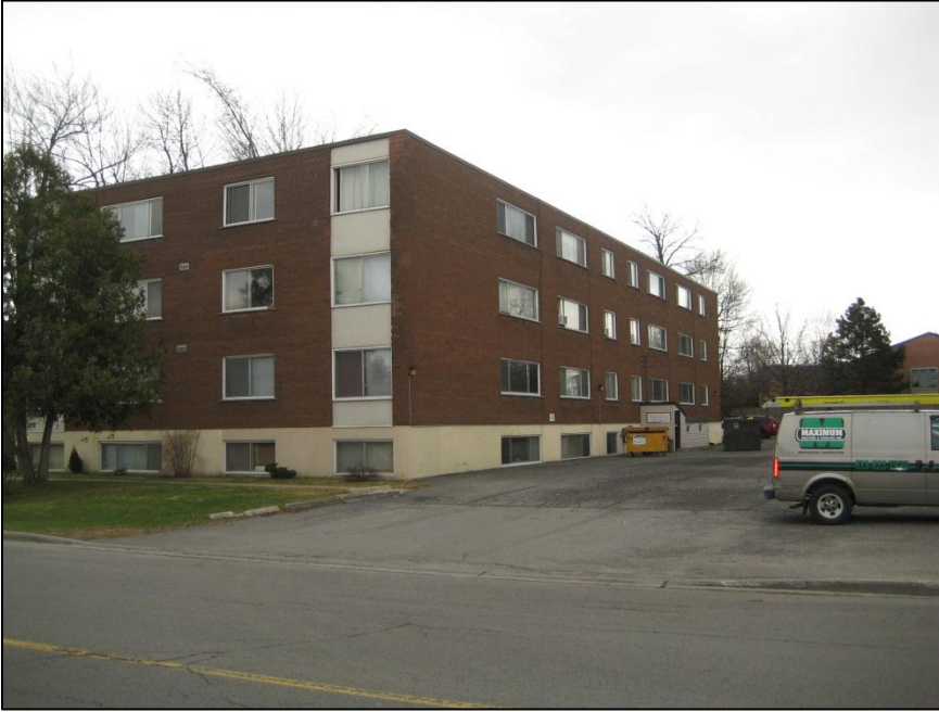
Photo No.1: View of the Site from Coronation Avenue (facing south)
