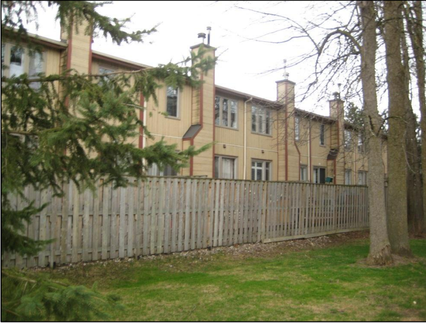
Photo No. 9: View of eastern neighbouring property (facing southeast)
