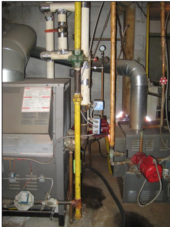
Photo No.14: View of the furnace room
