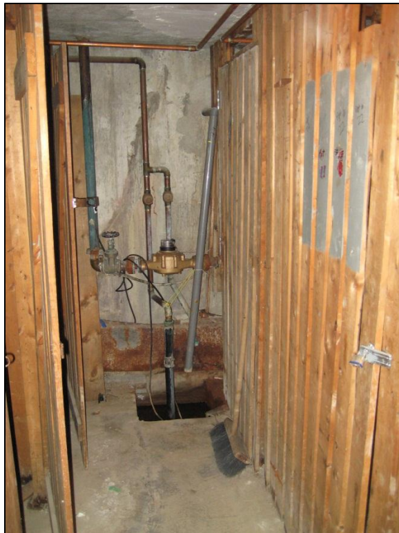
Photo No.20: View of basement with sump
