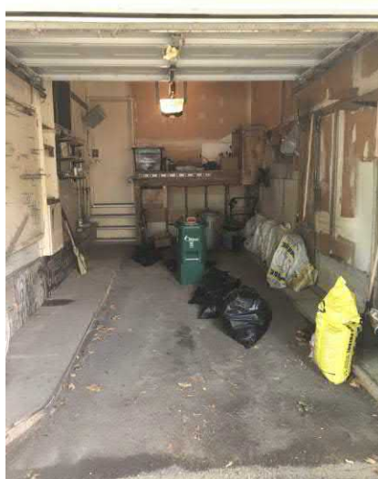
Photo 20: Garage at 810 Vick.
