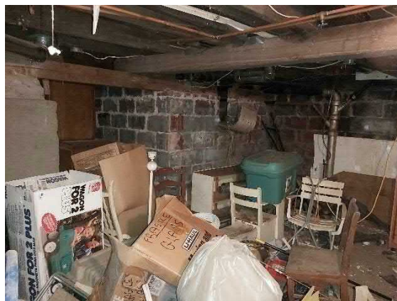
Photo 4: Basement of 2830 Carling.
