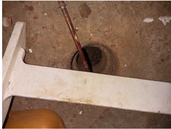
Photo 6: Drain in the basement of 2830 Carling Ave
