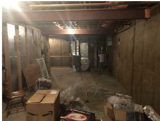
Photo 17: Basement of 810 Vick.
