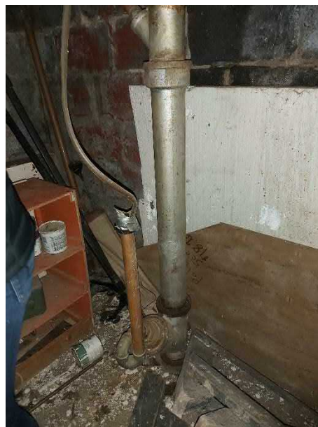
Photo 5: Pipe in the basement of 2830 Carling.
