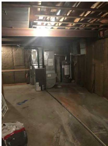
Photo 14: Basement view of 810 Vick.
