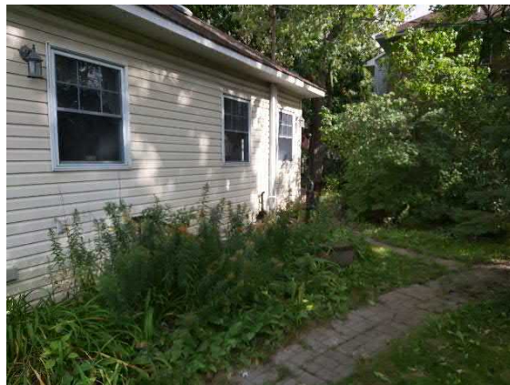
Photo 8: Front exterior of 2830 Carling.
