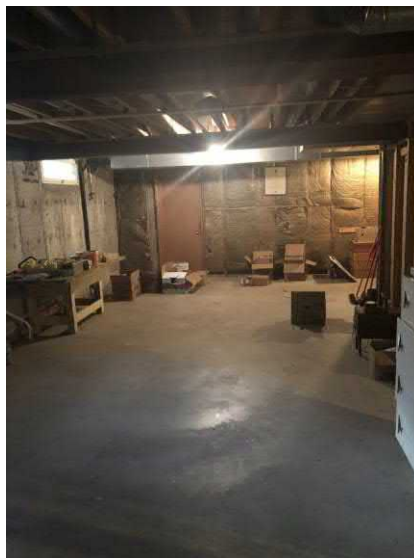
Photo 19: Basement of 810 Vick.
