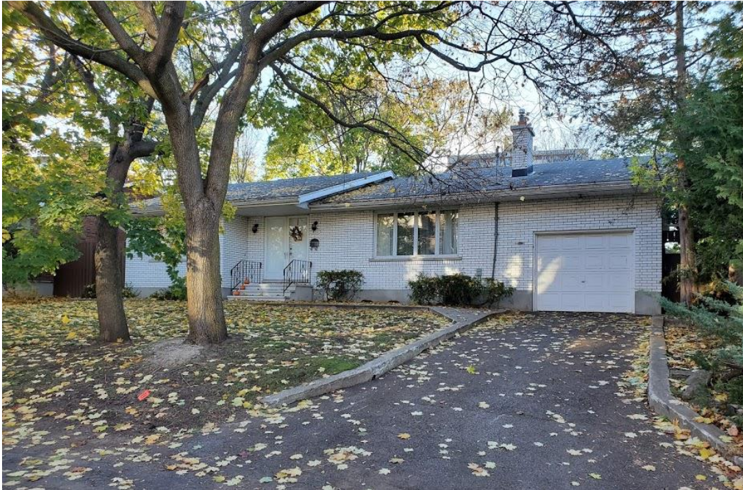
Photo 9: 810 Vick Avenue which forms part of the Subject Property
