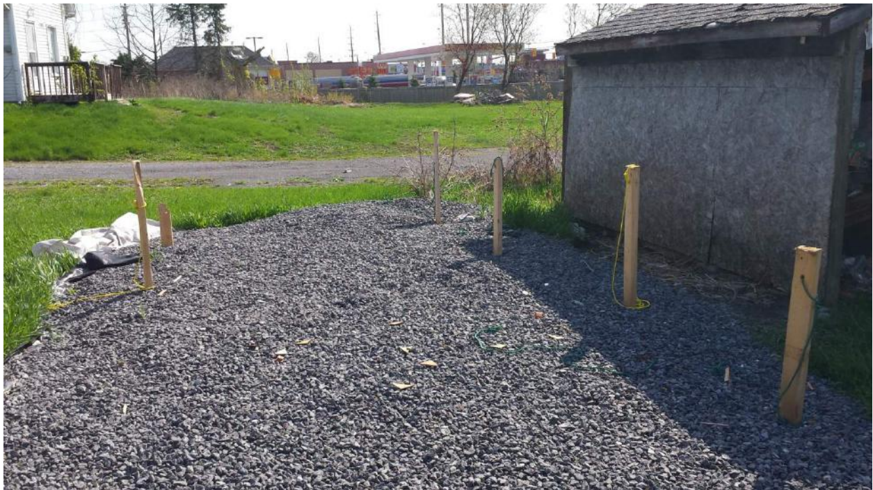
Photograph 6: Gravel pad and shed at 3835 Innes Road, looking east. The building at 3843 is visible at top left, and the adjacent retail fuel outlet at 3869 Innes Road is visible at the top.
