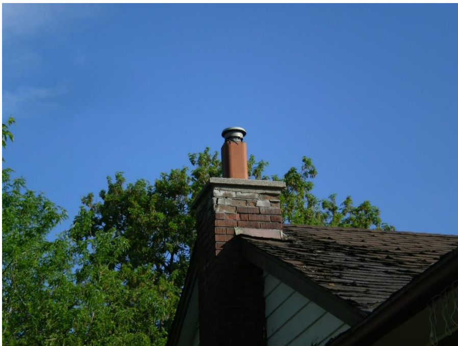
Photo 6 – Chimneys on the central and west residences are vented. This example is on the residence in the northwest portion of the site. View looking north
