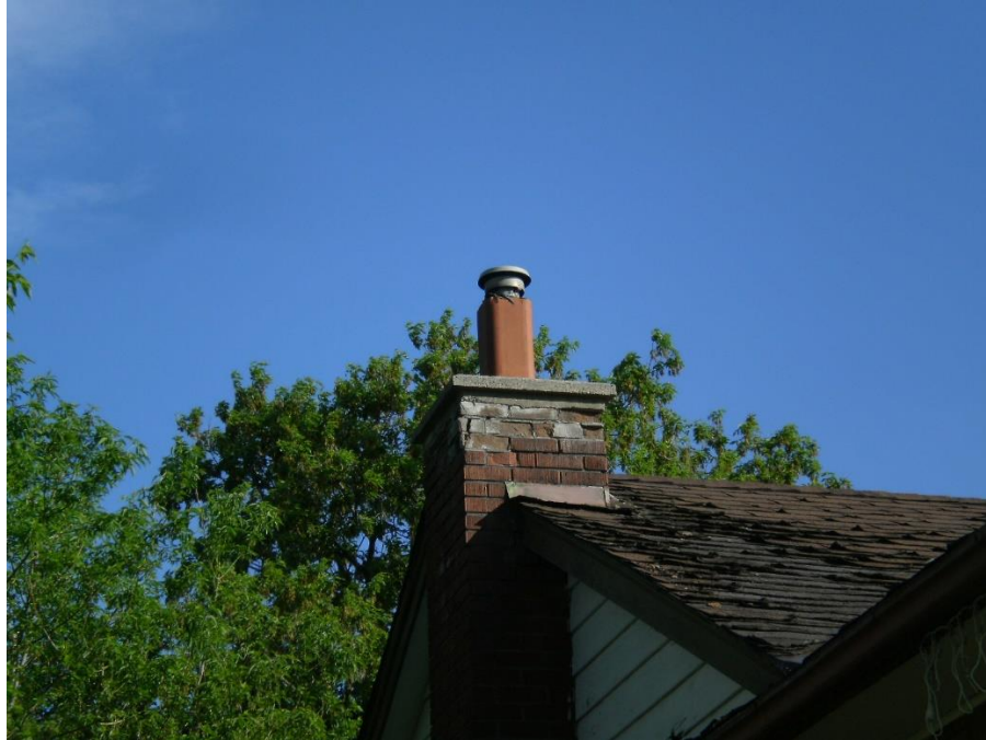
Photo 6 – Chimneys on the central and west residences are vented. This example is on the residence in the northwest portion of the site. View looking north
