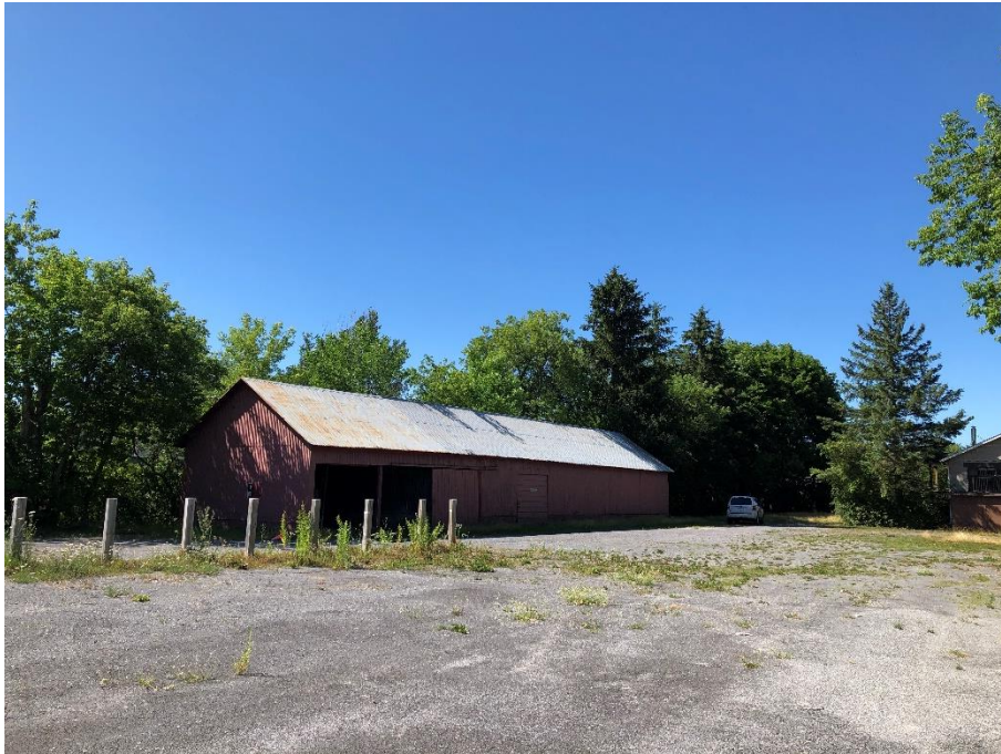
Photograph 1: Photograph illustrates the existing workshop/garage located at 1518 Stittsville Main Street of Phase I Property, facing southwest.
