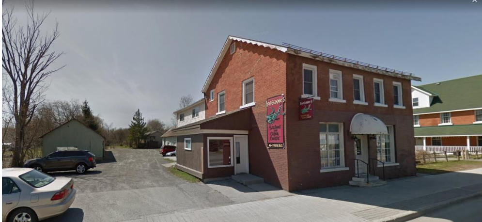
Figure 4: 1518-1526 Stittville Main Street, 2012, prior to the fire in 2013 that led to the demolition of the building and its rear extensions. The front verandah had already been removed by this time, possible to allow for the widening of the sidewalk. Source: Google Streetview, image capture April 2012.
