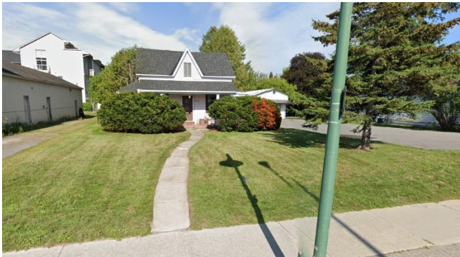
Figure 15: 1543 Stittsville Main Street (further right building), located about 100 m and across the street from 1518 Stittsville Main Street. Source: Google Streetview, September 2019.
