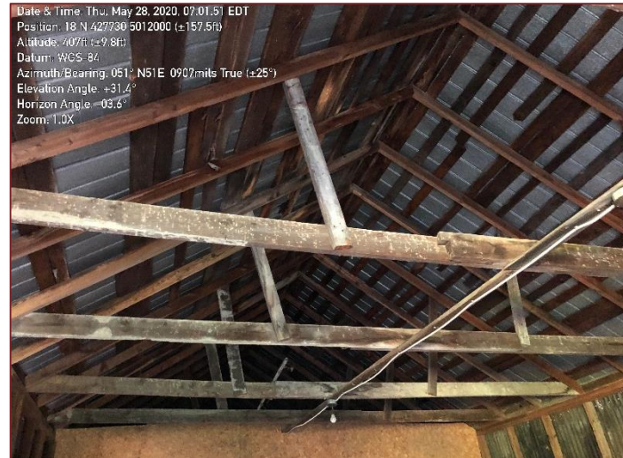
Site Photograph 4 – Inside Roof of Barn Structure
