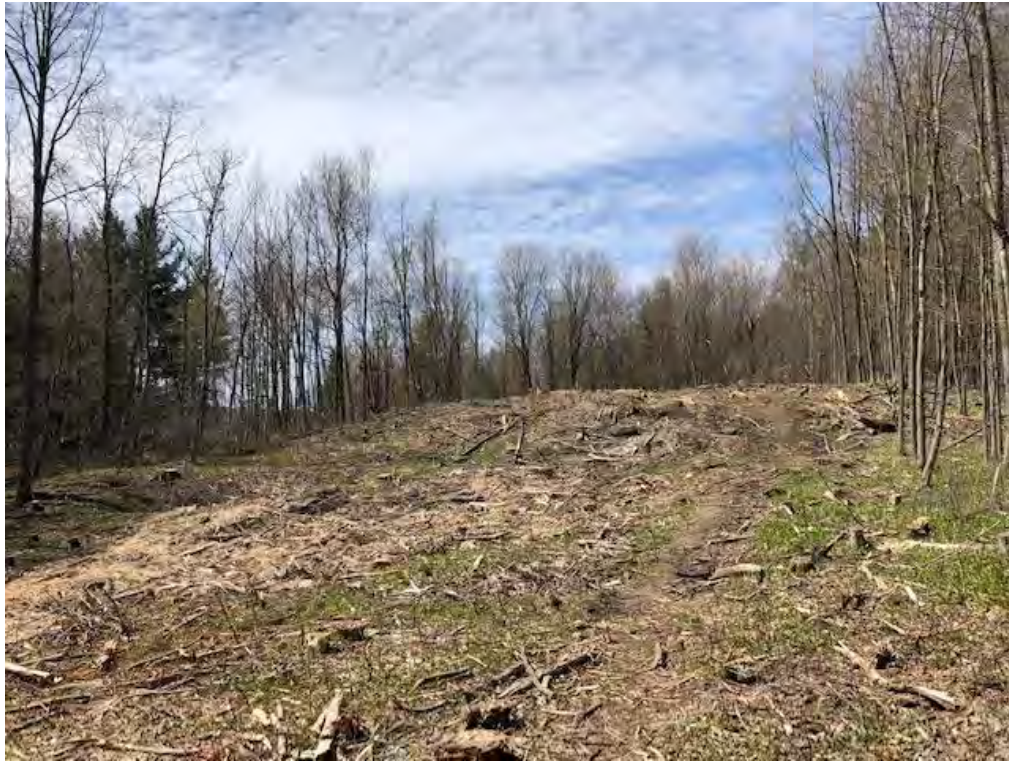
Photo 1: May 14, 2020. Clearing of FODM5-4 to accommodate Canadian Shield Avenue extension.
