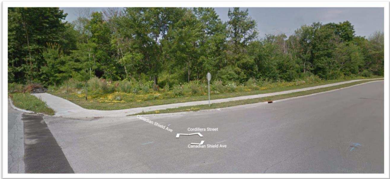
View looking west at subject property from Cordillera Street at Canadian Shield Avenue
