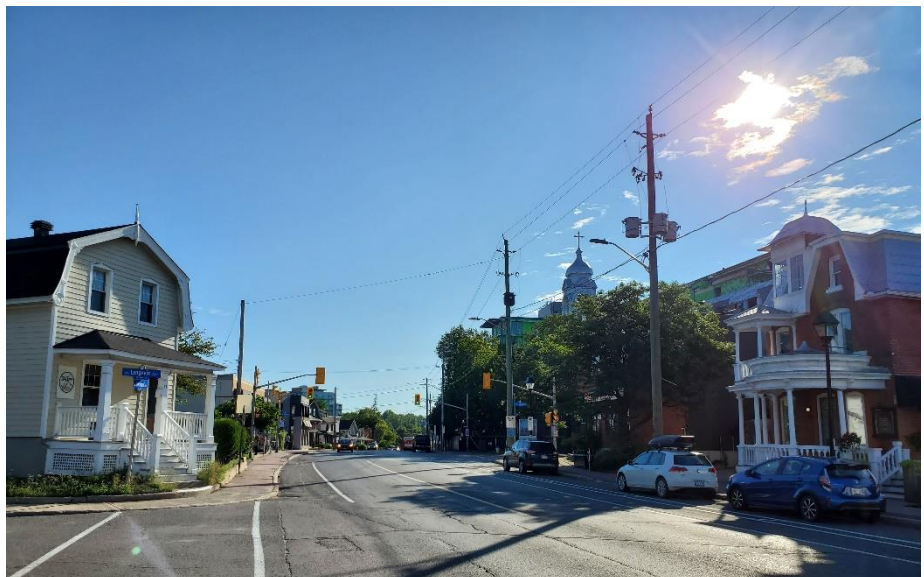
29 81 Beechwood Facing 98 Beechwood Heritage Properties with the domed bell tower of the Former St. Charles Church visible in the background. MTBA
