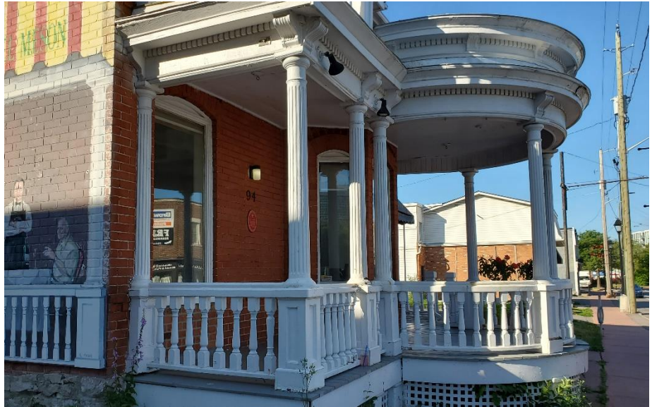
28 Detail of the porch on 98 Beechwood Avenue. MTBA
