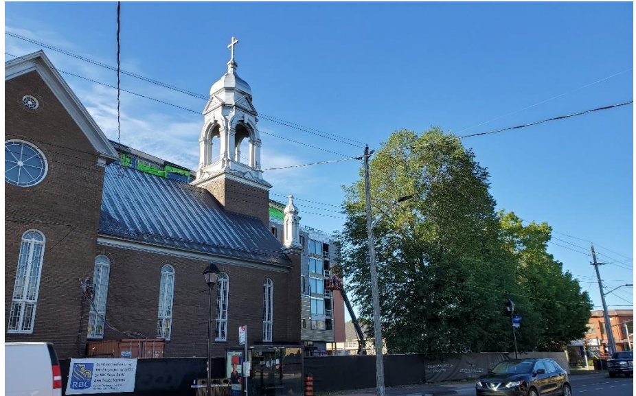
33 Looking southwest along Beechwood Avenue towards the former St. Charles Church with a new development visible beyond. MTBA
