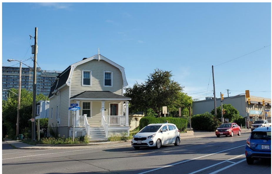
24 81 Beechwood Avenue with immediate context. MTBA
