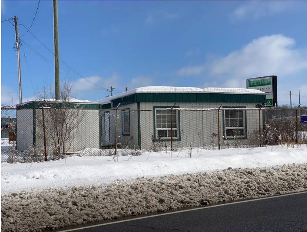
Photo 3: View of the temporary building located at the Site
