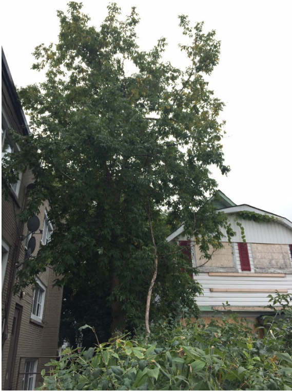
Figure 2: Tree 1 - Manitoba maple right beside excavation and where new building will be
