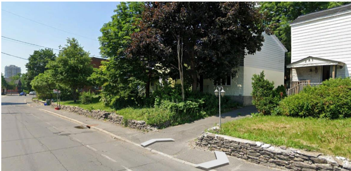
Figure 16: Street view looking south on Beechwood. 247 Beechwood is to the right, and the roof of 231-235 Beechwood is visible to left. Note the stone retaining wall at the street, and the simple landscape treatment. Source: Google Earth
