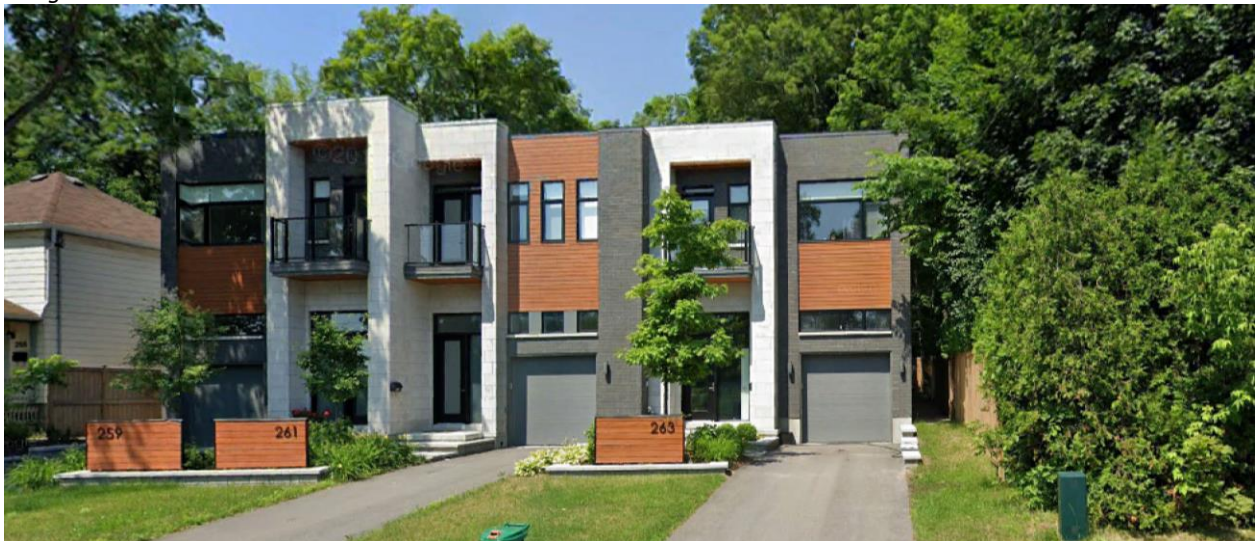
Figure 8: Street view of 259, 261, and 263 Beechwood Avenue to the north of Corona Avenue, a recent development within the HCD. Source: Google Earth
