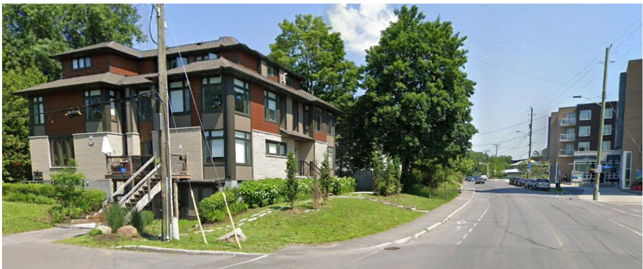
Figure 6: Street view looking north. The property at the corner 455 Green Avenue (left) is an example of recent development in the Panhandle of Rockcliffe Park. Source: Google Earth
