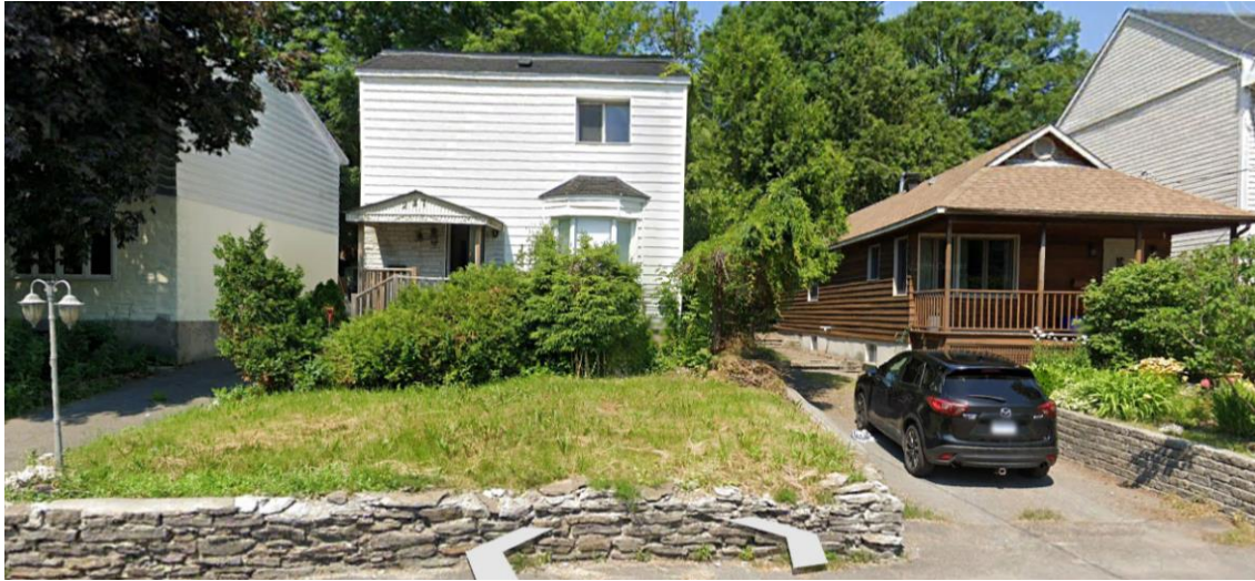
Figure 15: Street view of the circa 1950 two-storey single detached properties at 245 (left), and 247 (centre) Beechwood Avenue built to standard plans developed by the CMHC. The small cottage-style residence at 249 (right) Beechwood is not part of the proposed development. Note the stone retaining wall at the street, and the simple landscape treatment. Source: Google Earth
