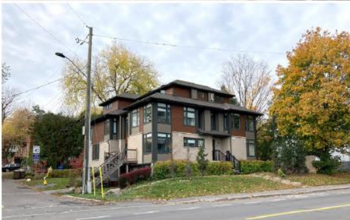
2: Street view looking north at the corner of Beechwood ave. and Green ave. 455 Green avenue. is an example of recent development in the area.
