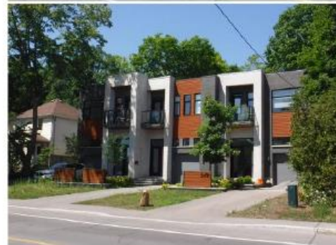
7: Street view of the recent development 259, 261, and 263 Beechwood ave. to the north of Corona ave.
