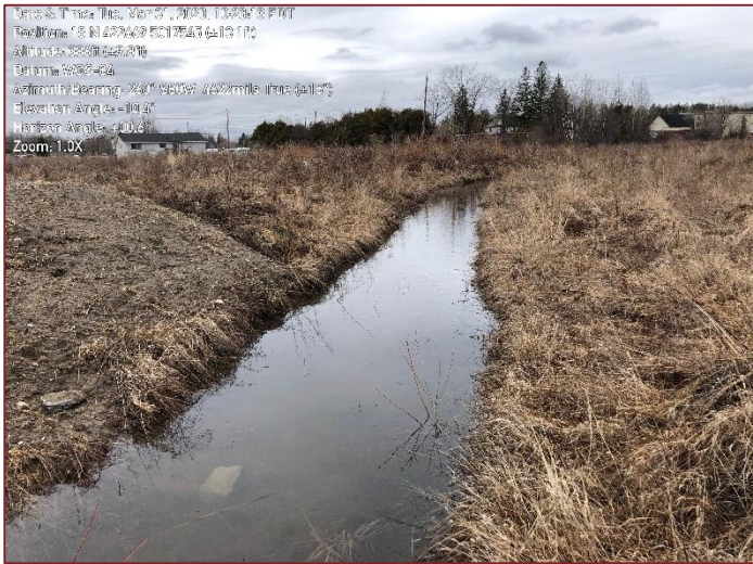
Site Photograph 1 – HDF1-1A looking downstream (March 31, 2020)
