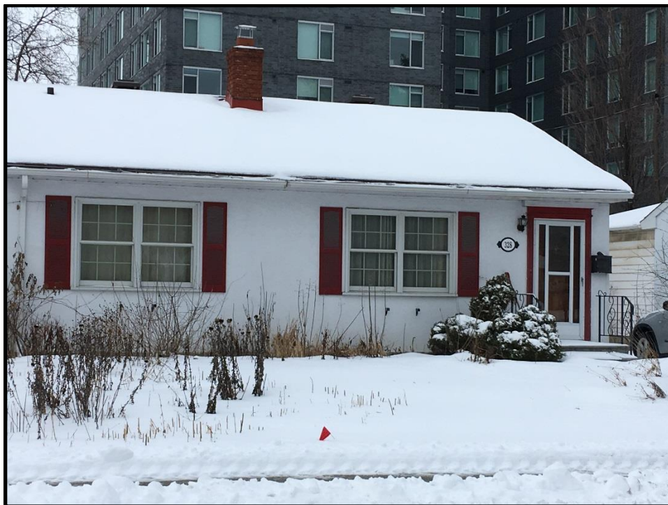
Photograph 4: East face of subject building addressed 328 Clifton Road, looking west.
