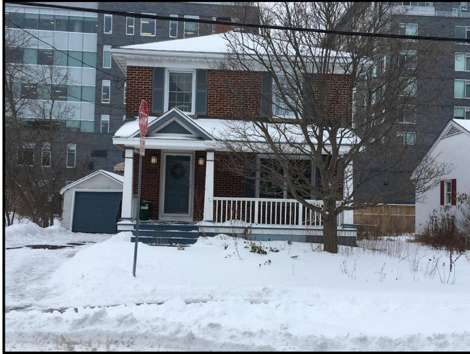
Photograph 5: East face of subject building addressed 332 Clifton Road, looking west.
