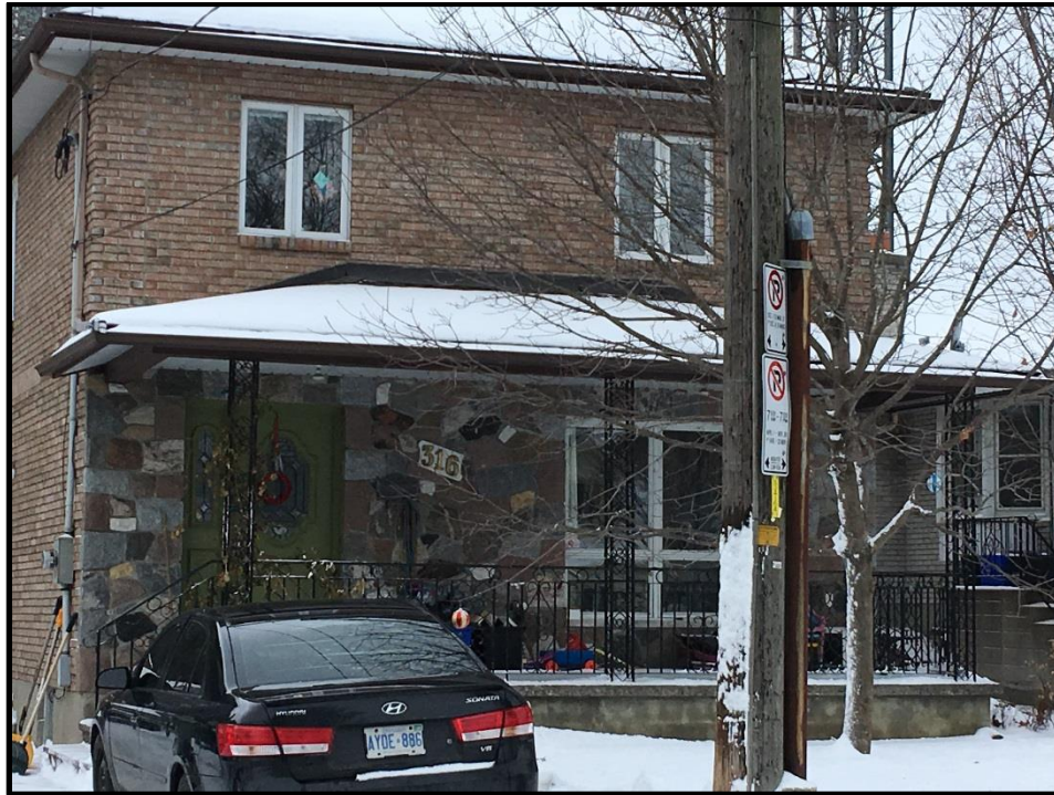
Photograph 1: East face of subject building addressed 316 Clifton Road, looking west.
