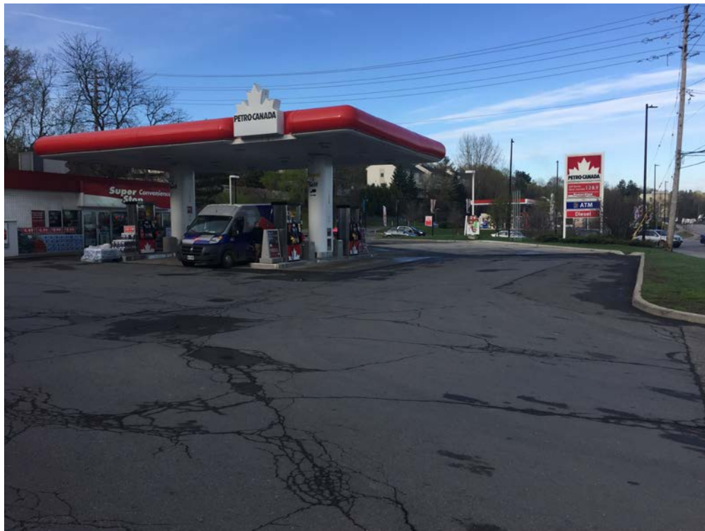
Existing Fuel Service Station located immediately west of site
