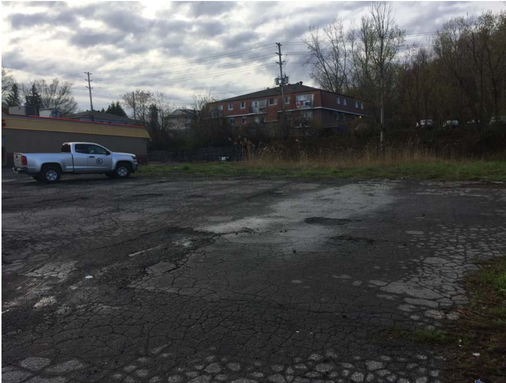
View of Site facing south
