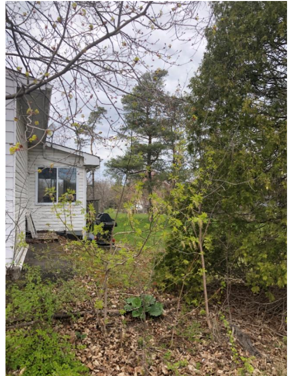
View looking at rear side Property
