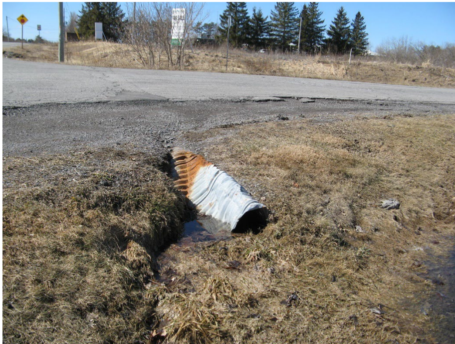
Photo 6 – Downstream end of culvert on the east side of John Cavanaugh Drive is damaged and there is no connection to the swale on the north side of McGee Side Road. View looking west
