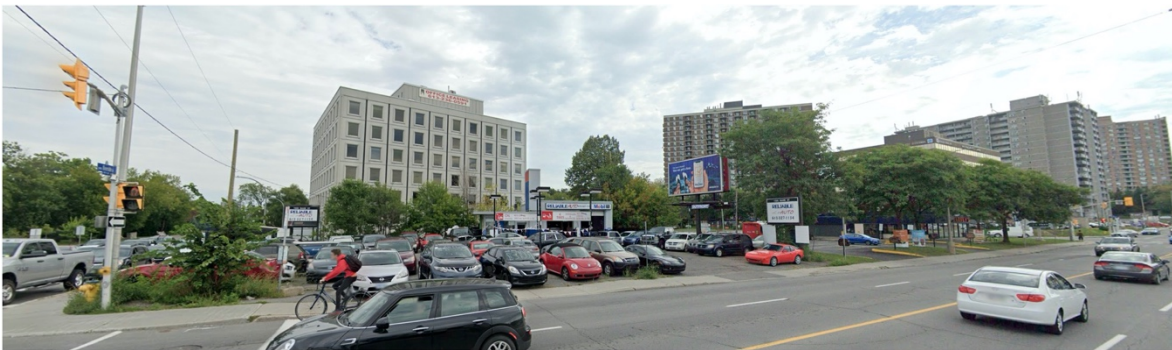
Figure 4: View of site from Bank Street looking northeast at site
