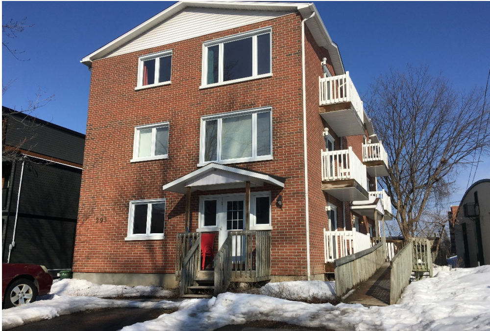
Photograph 1: View of south face of 295 Ashton Avenue, looking northwest.
