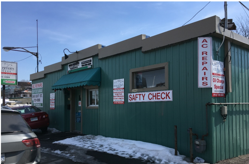
Photograph 6: View of northeastern portion of the Phase I Property, facing southeast. Photograph illustrates the north face of the automotive service garage at 2046 Scott Street.
