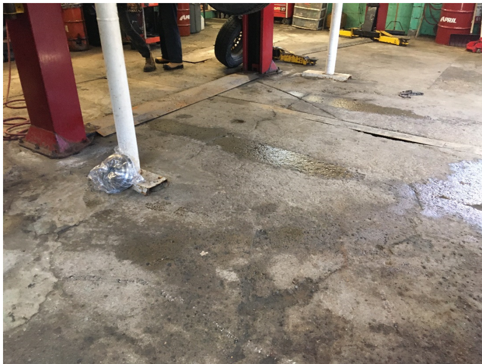
Photograph 10: View electric hoist and floor drains on the interior of 2046 Scott Street.
