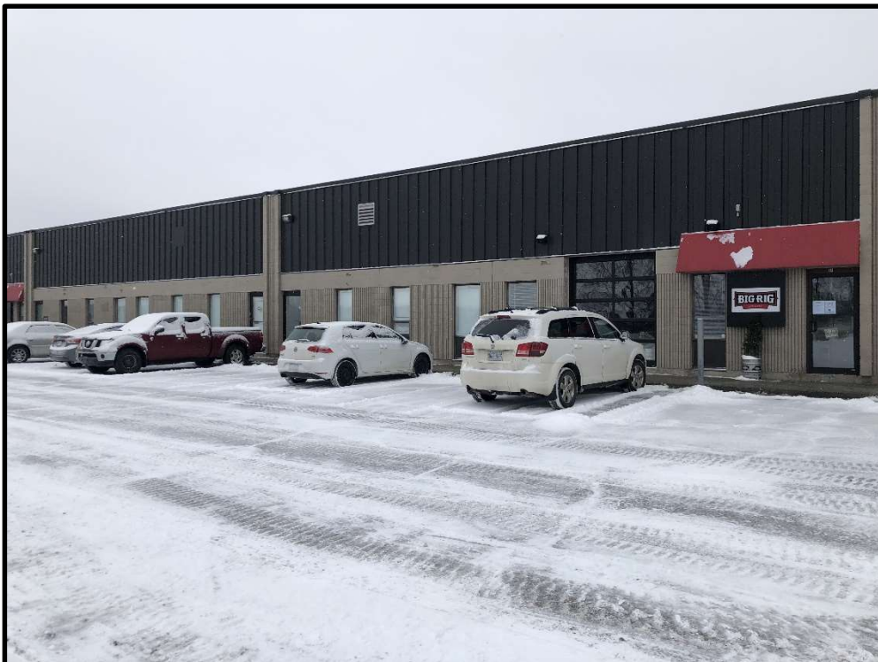
Photograph 2: Front view of 101 (A), looking southeast.
