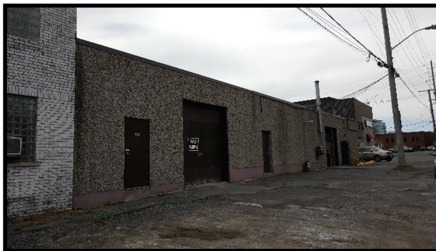
Photograph 4 – View of a portion of the west elevation of the Site building associated with 951 Gladstone Avenue.
