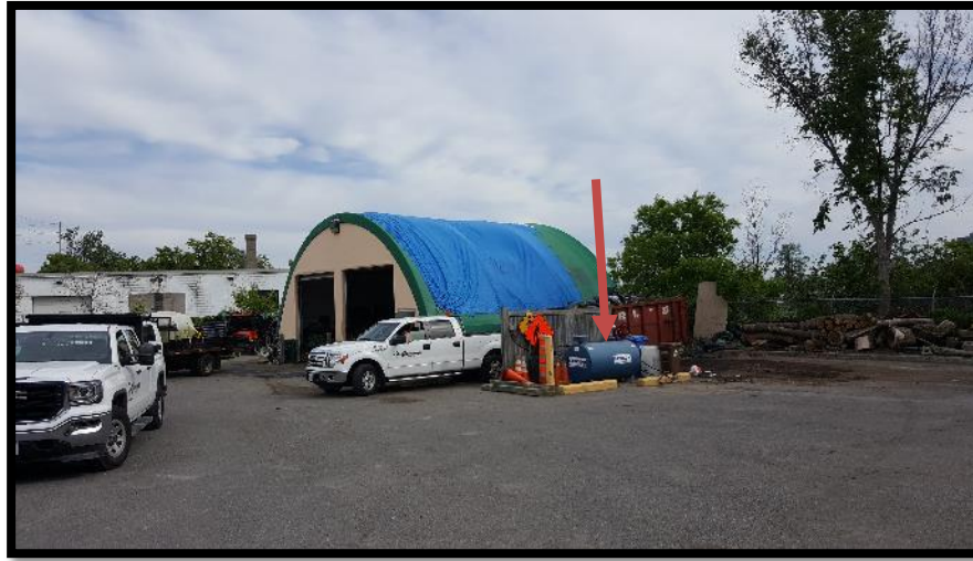
Photograph 7 – View of the gasoline AST (see arrow) on the northeast portion of the Site.
