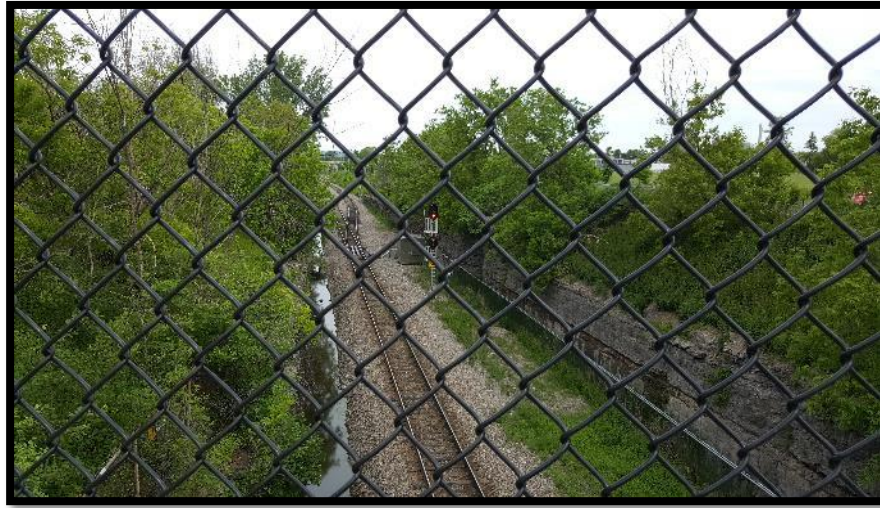
Photograph 9 – View of a portion of the adjacent railway corridor to the east of the Site..
