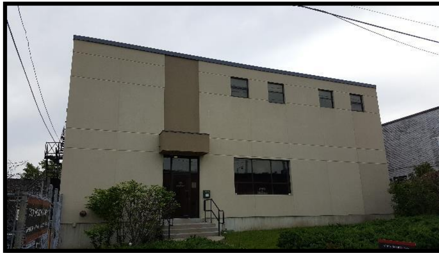
Photograph 6 – View of the west elevation of the Site building associated with 145 Loretta Avenue North.
