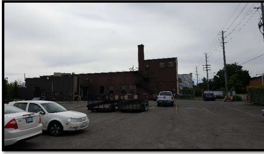
Photograph 5 – View of the north elevation of the Site building associated with 145 Loretta Avenue North.
