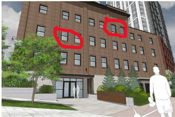
Figure 24 and 25: The fenestration along the east facade follows the profile of the original building as the as-found drawing below illustrates. Highlighted in red are proposed windows replacing doors and the introduction of new windows that were not originally part of the façade.
