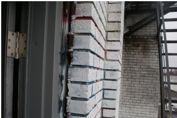
Figure 32: View of the exterior brickwork from a second-floor fire escape. Note the highly textured brick surfaces and recessed joint profile. Source: Commonwealth 2020.
